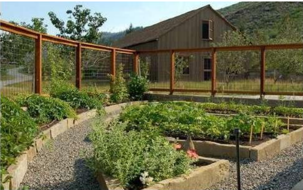
Welded mesh garden fence.
