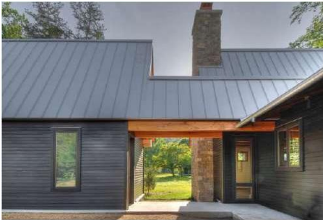
Wood siding oriented horizontally.
