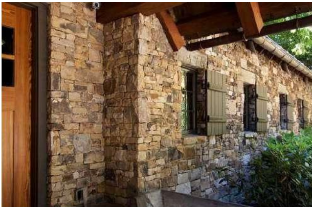
Indigenous dry stack stone exterior.
