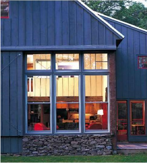
Fiber cement board siding with vertical battens.
