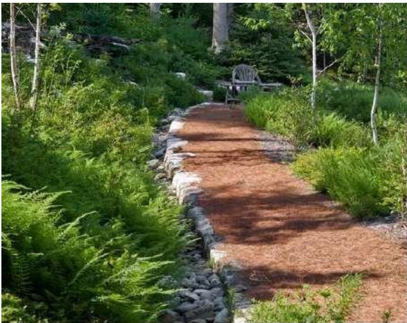
Infiltration trench paralleling a pathway.
