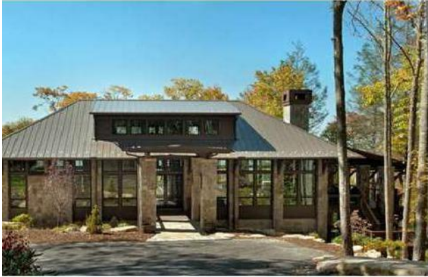
Standing seam metal roof with low sheen.
